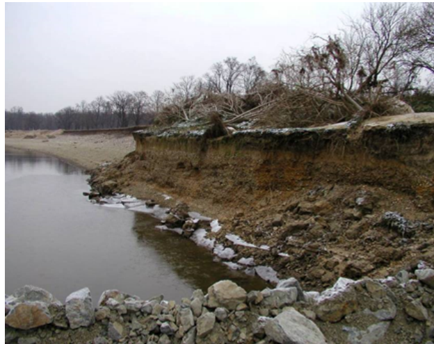
Damaged Vltava river bed and banks after 2002 flood
