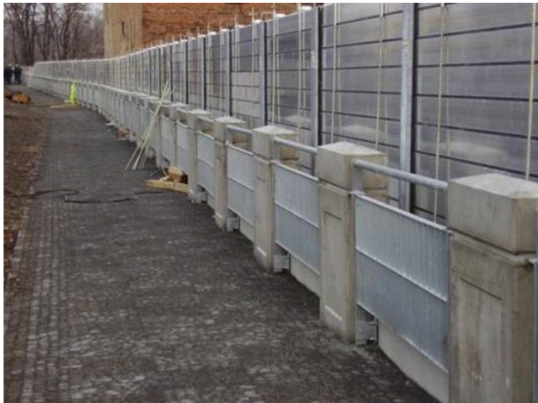
Erected temporary flood barriers in Prague-Holešovice
