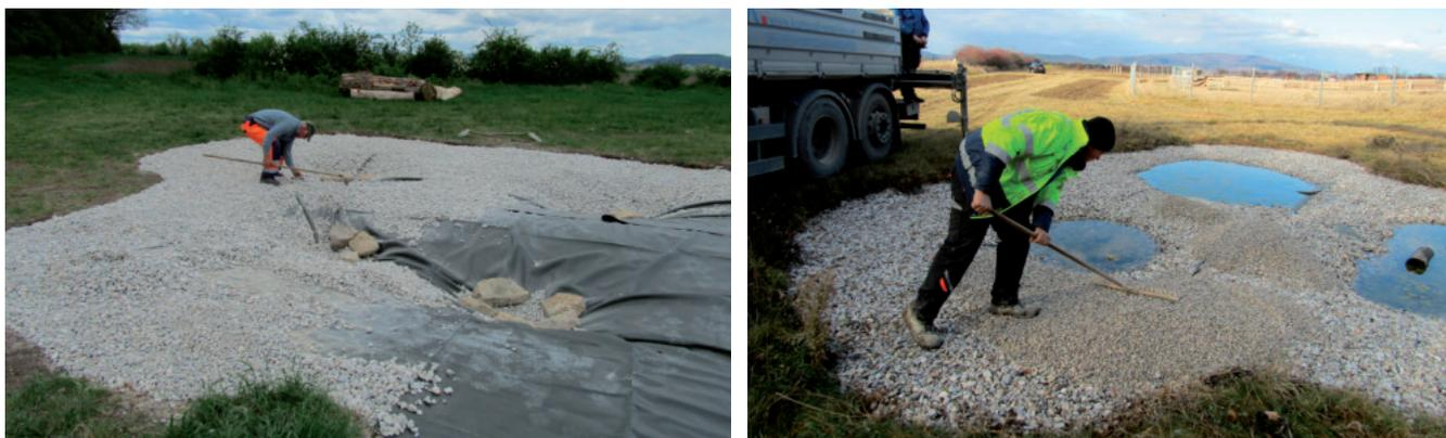
*Fig: Building of a pond. The pond is sealed with pond liner.*
